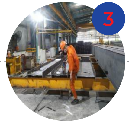
3 KHOAN LỖ Drilling
