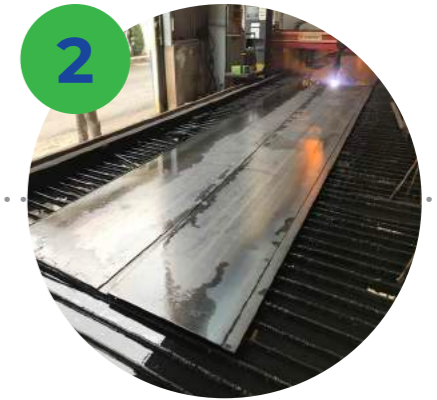
2 CẮT THÉP TẤM Cutting/shearing
