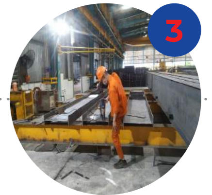
3 KHOAN LỖ Drilling
